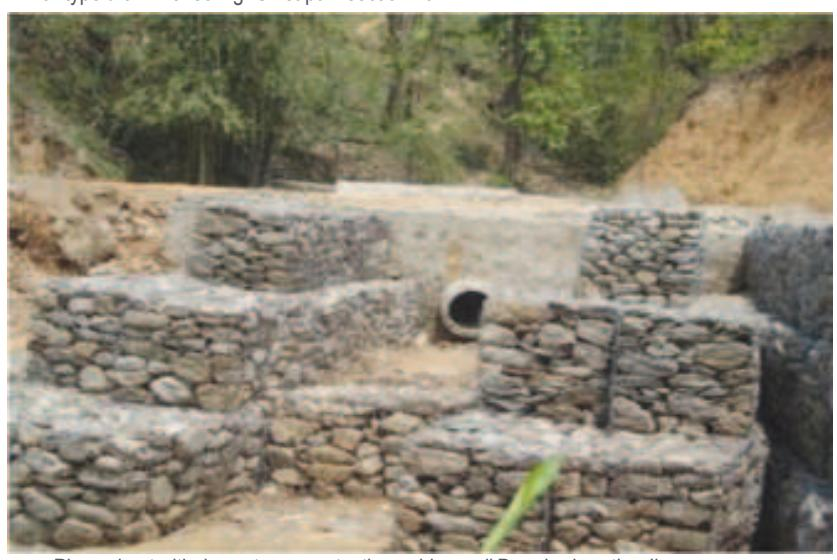
Pipe culvert with downstream protection gabion wall Danabari section-llam
