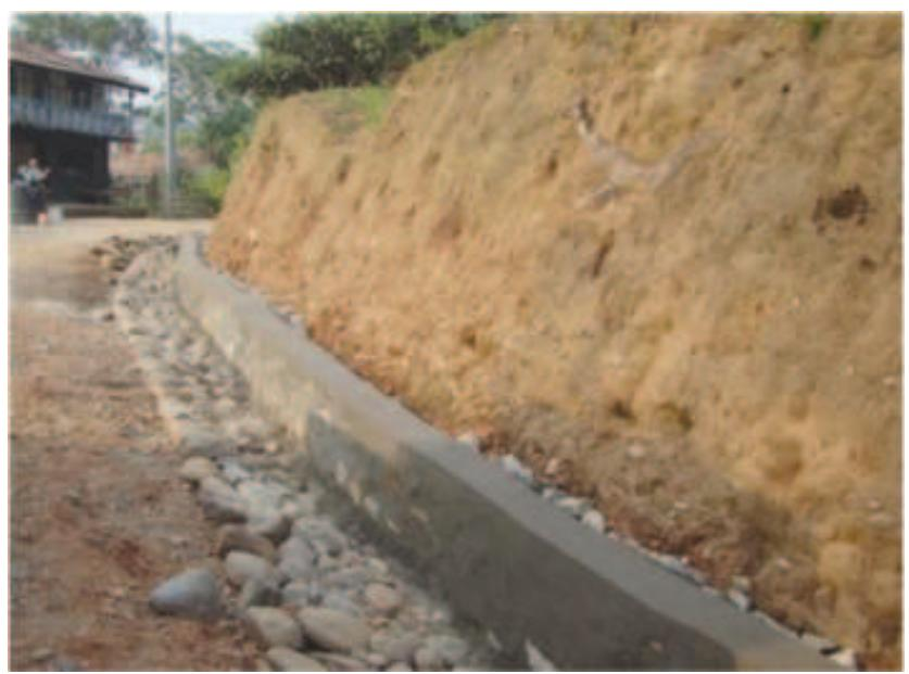
Tick type drain with soling- Chisapani section-llam
