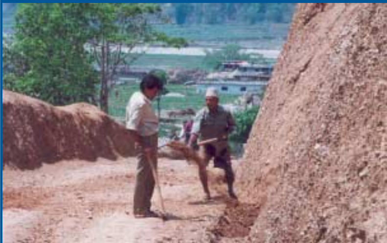
Figure 14: Implementing rural access improvement works
