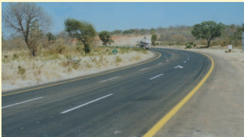
After some months the Otta Seal with a sand cover seal are fully settled and shows excellent appearance. (Botswana).
