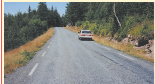
Otta Seal using crushed aggregate on a primary road after 6 years in service. (Norway).
