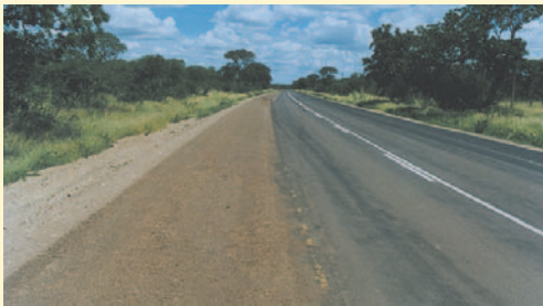
An Otta Seal will apparently show a significant difference visually between the shoulders and the carriageway. The traffic in the carriageway area works the binder upwards to the surfacing and hence, making difference in colour. This difference in colour will improve the traffic safety aspect. (Botswana).
