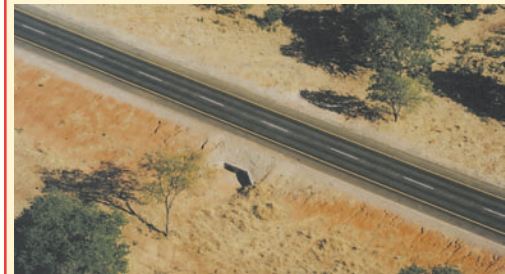
The same road in a “bird view”. Note the appealing uniform appearance, more like an asphaltic concrete. (Botswana).
