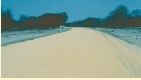
Over application of sand is essential when applying a sand cover seal on top of a single Otta Seal. (Botswana).
