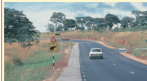
A bituminous surfacing protects the base course layer and provides good riding quality. Hence, low operational costs. (Zimbabwe).
