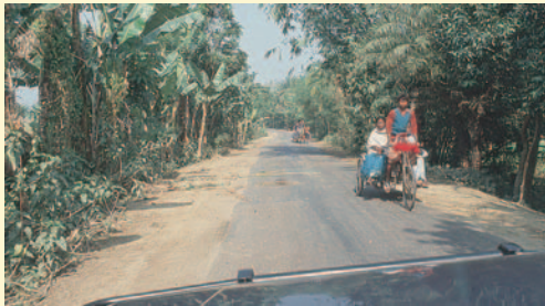
The final product, a Single Otta Seal after 2 years in service. (Bangladesh).
