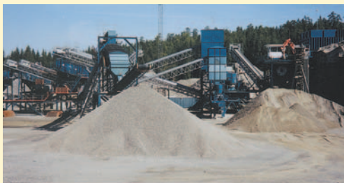
Sophisticated and expensive crushing plant is normally required to produce aggregate for Chip Seals. (Norway).
