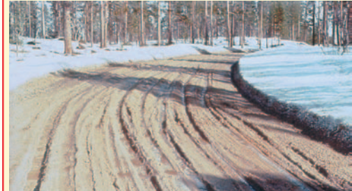
The unpaved road network was in a poor condition in Norway in the early sixties. During the thaw period often un-passable for both light and heavy vehicles. (Norway).
