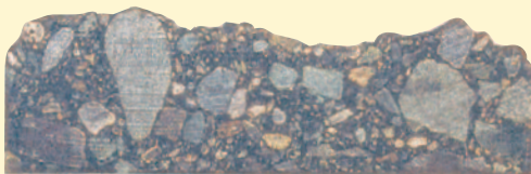
The mechanical interlocking, and bitumen binding of the Otta Seal is "a bit like" bituminous premix. A Double Otta seal.
