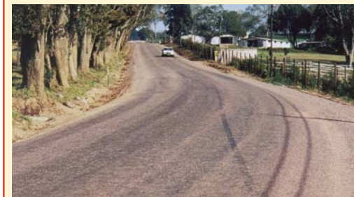
The same road as above, but after 3 months in service. (South Africa).
