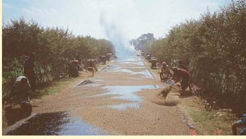
The Otta Seal aggregate was applied by labour based methods, by pre-stockpiling the hand crushed aggregate. A 100 metre long section, 3,7 metres wide was covered by aggregate after 7 minutes time, and the section was opened to traffic. (Bangladesh).
