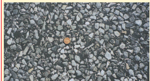
Close-up of the Otta Seal surfacing. (Norway).
