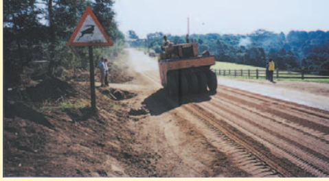
Extensive rolling with pneumatic rollers is essential to achieve a good result. (South Africa).
