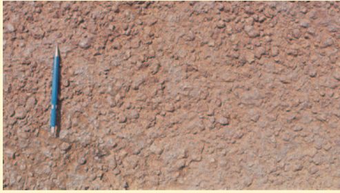
Close-up of an Otta Seal where natural occurring laterite was used as Otta Seal aggregate. (Kenya).
