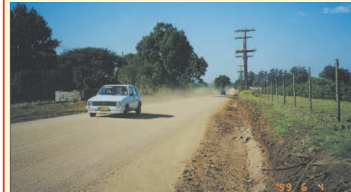
Unsealed roads very often provide an unsatisfactory driving comfort and associated high maintenance and operational costs. Dust pollution is also a problem in urban areas. (South Africa).
