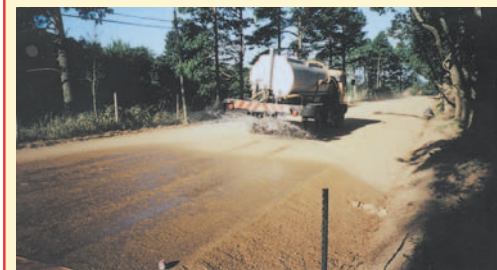
Light watering of the broomed base before spraying the binder will enhance the bond between the base and the Otta Seal. (South Africa).
