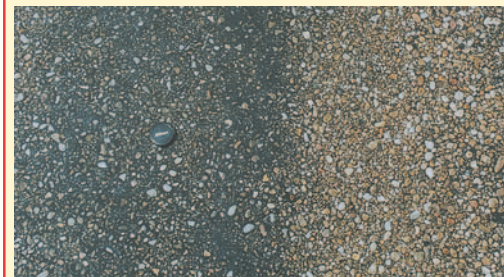
Close-up, after 8 - 10 weeks the aggregate beds down. (Botswana).
