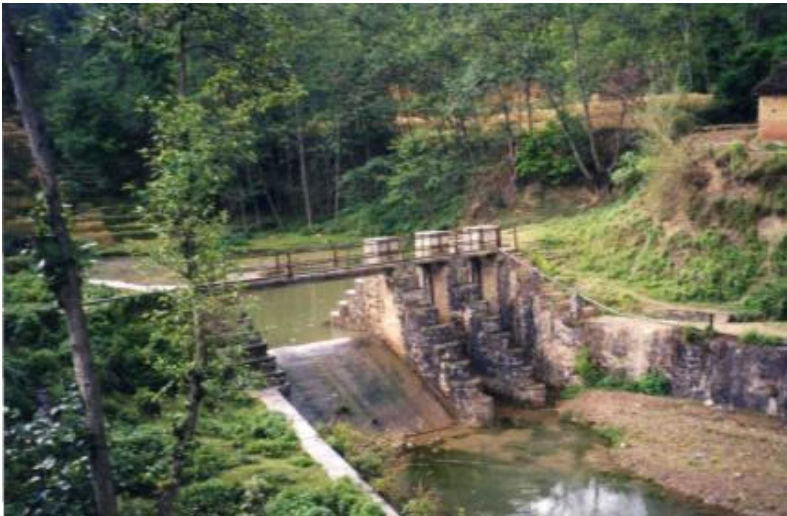
Figure 4-4: Concrete weir and undersluice
