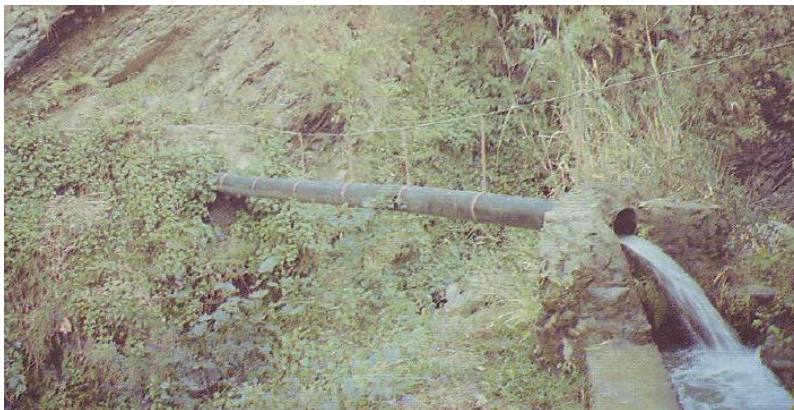
Figure 8-4: HDP Pipe Crossing
