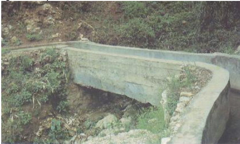
Figure 8-1: Aqueduct in Hills
