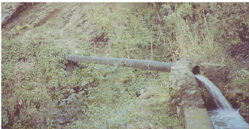
Figure 8-4: HDP Pipe Crossing
