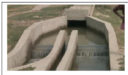
Figure 7-1: Definition Sketch and Photograph of Proportional Divider
